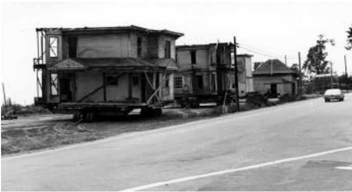
The house, carriage barn and water tower ready for move to Centennial heritage Museum
