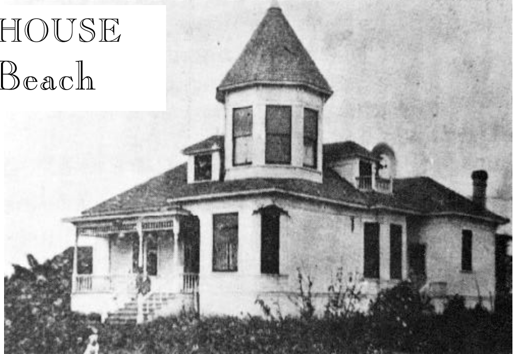
Earliest known picture of the Newland house in Huntington Beach, pre 1912
